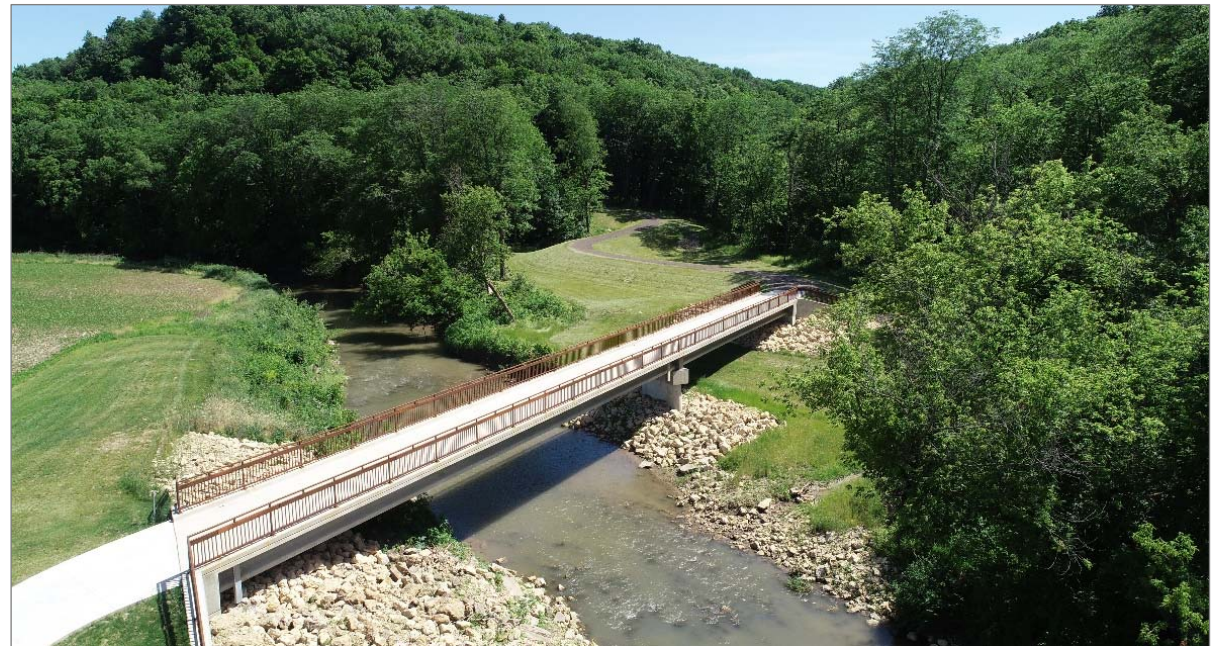
Felderman Park Pedestrian Bridge over Mill Creek (Source: Bellevue Video LLC)
