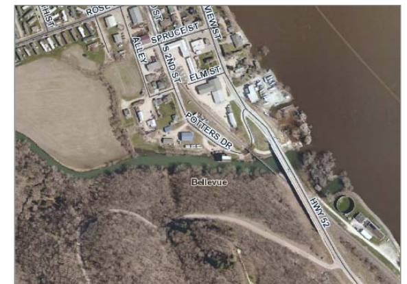
US Highway 52 Bridge south (Source: Jackson County GIS)
