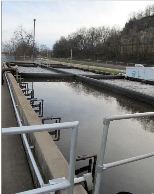
Bellevue Wastewater Treatment Plant (Source: City of Bellevue)
