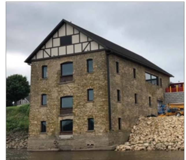
Water Street Landing, 305 S Riverview St. $1.8 million renovation of historic button factory completed in 2020 for office and retail space, business incubator, center for school and civic programs, public restrooms, public dock amenities, and parking. (Source: ECIA)
