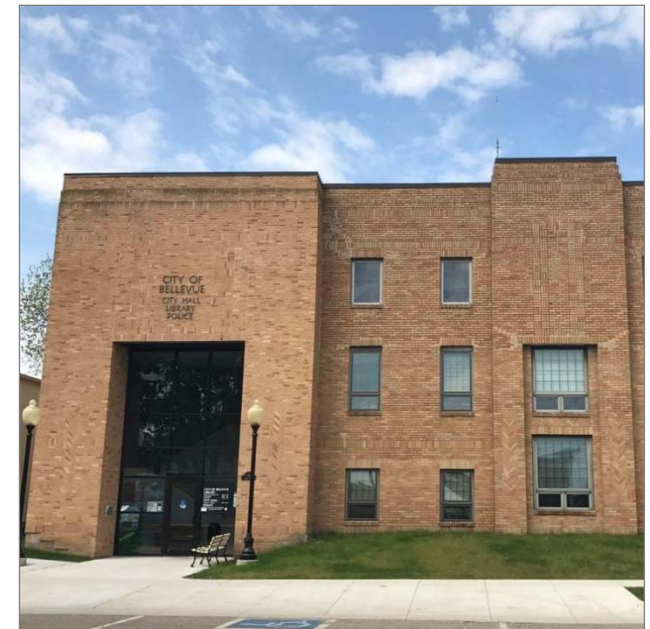
Bellevue City Hall, Public Library, and Police Department (Source: City of Bellevue)
